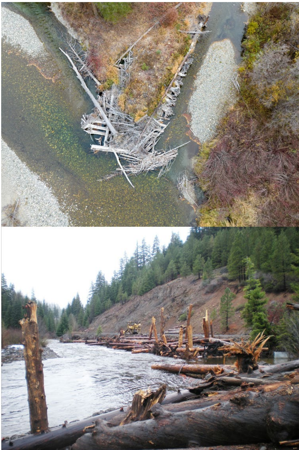
Figure 44. Example of a flow-splitting apex jam constructed on the Entiat River in central Washington State (top). Bottom photo shows wood bank revetment meant to protect the road from bank erosion while providing covered pool habitat.
