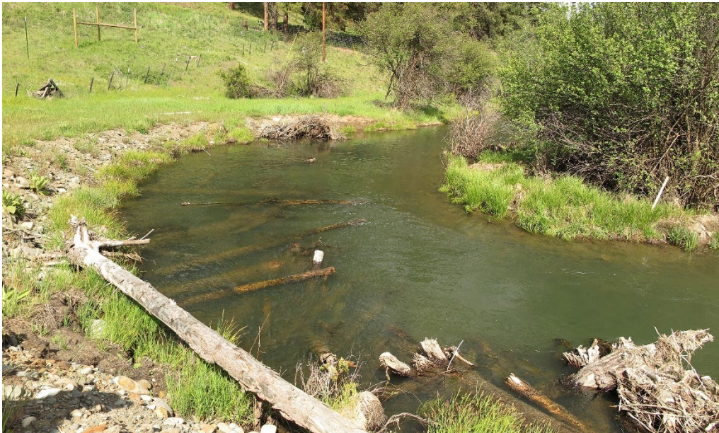
Figure 42. Example of pool excavation with wood loading to create holding and rearing habitat from the Middle Fork John Day River, OR.
