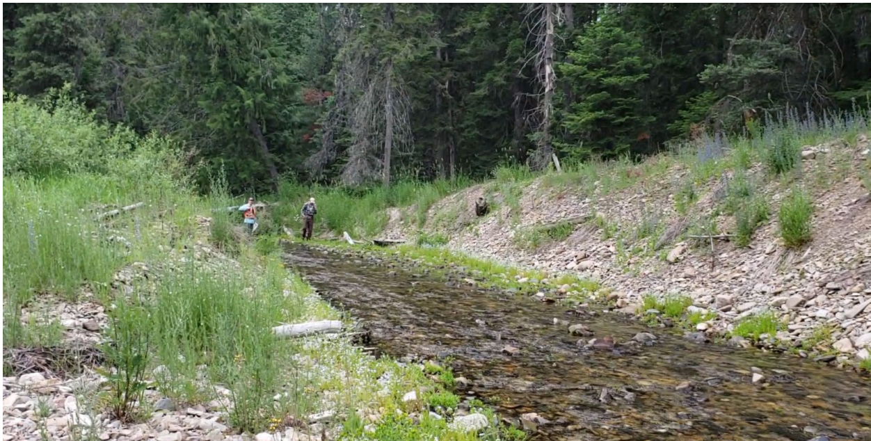
Figure 25. Photo looking downstream in the prominent side channel in Reach 3. Dredged material used to create a berm is visible on the right side of the photo (right bank).
